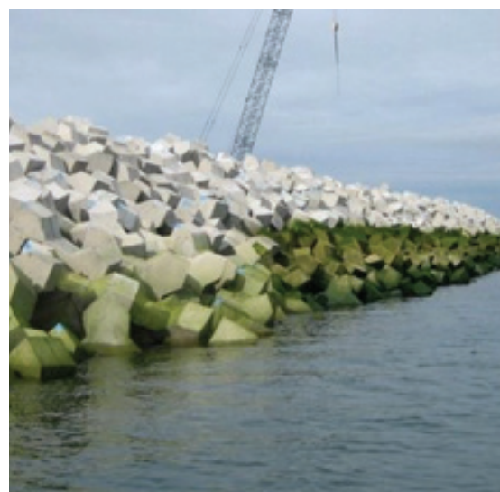
An example of a breakwater constructed using XBloc armour.
