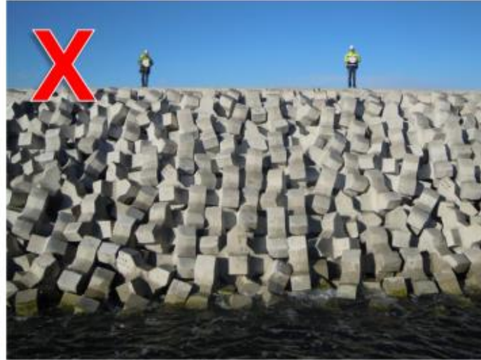
Xbloc units regular placement: High packing density
