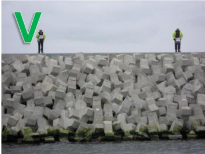
Xbloc units random placement: Good packing density
