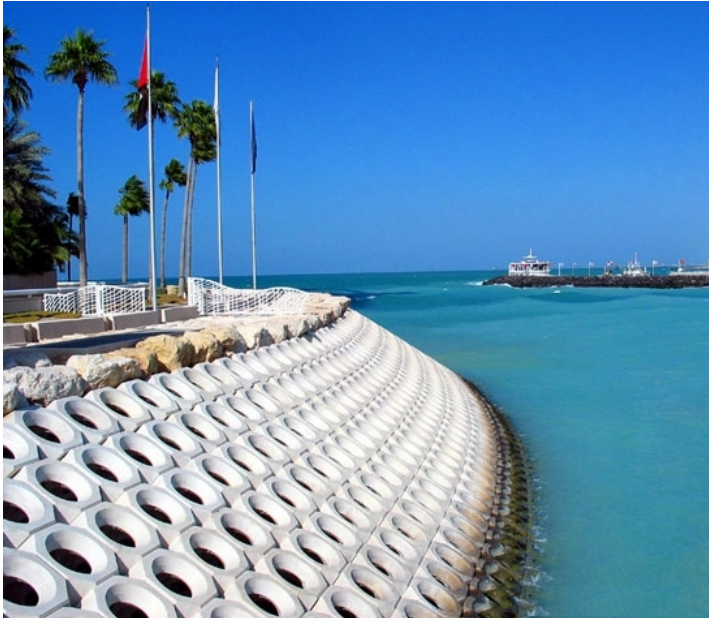
Figure 1: Shed armouring at Burj al Arab Hotel, Dubai, UAE
