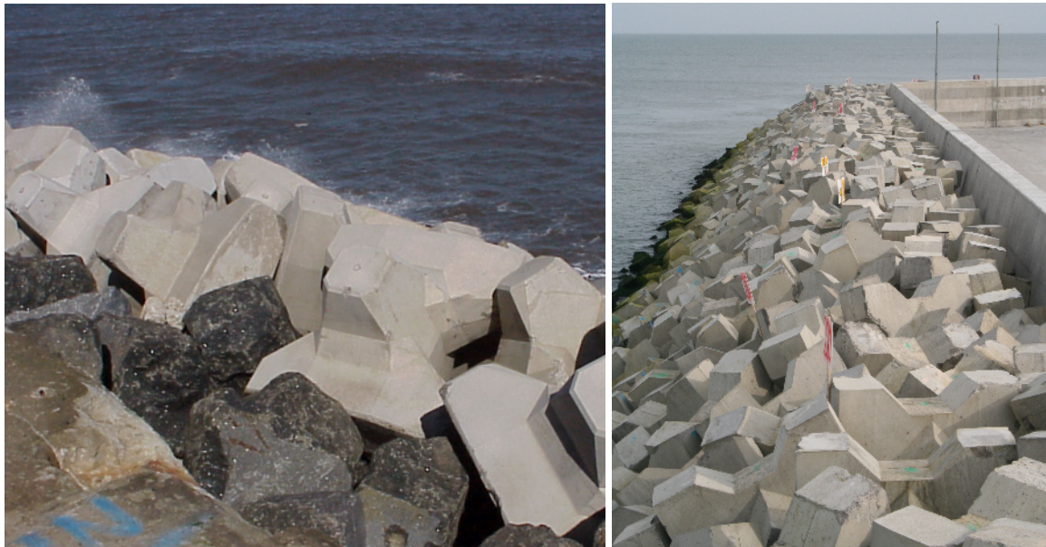
Figure 8: Single layer armouring: 6.3 m 3 Accropode™ (Scarborough, UK) and 4 m 3 Xbloc (Port Oriel, Ireland)
