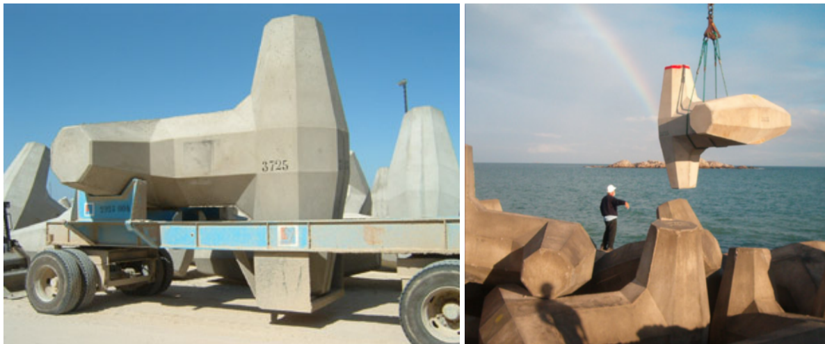
Figure 7: Transport and placement of Dolos units (30 t), Coega Port, South Africa
