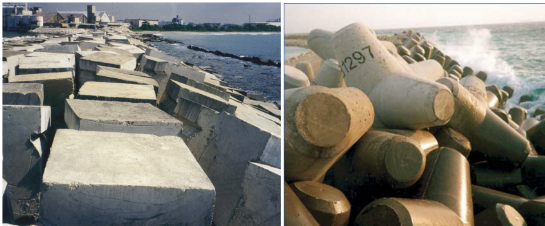
Figure 6: Double layer armouring: Cubes (left) and Tetrapods (right)
