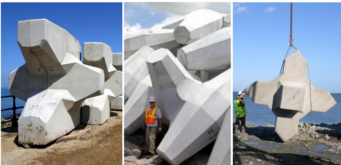
Figure 4: Single layer armour units: Accropode™ (6.2 m 3 , Scarborough, UK), Core-loc® (15 m 3 , Kaunapau Harbor, Hawaii) and Xbloc (4 m 3 , Port Oriel, Ireland)
