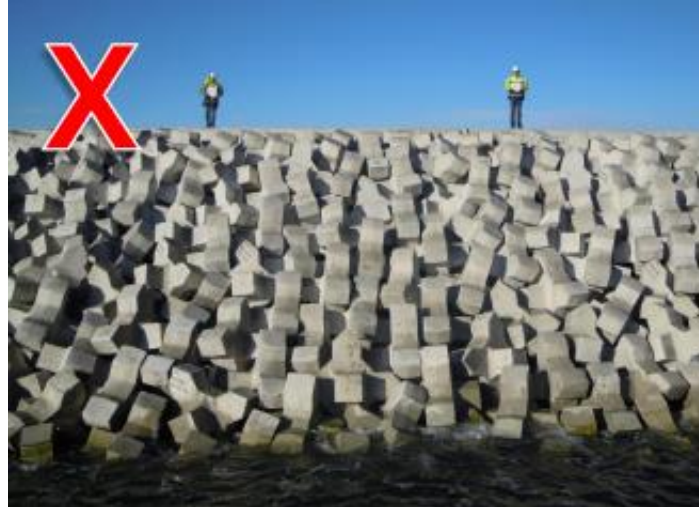
Xbloc regular placement: Higher packing density Faster placement (no thinking) Incorrect, but frequently seen in projects
