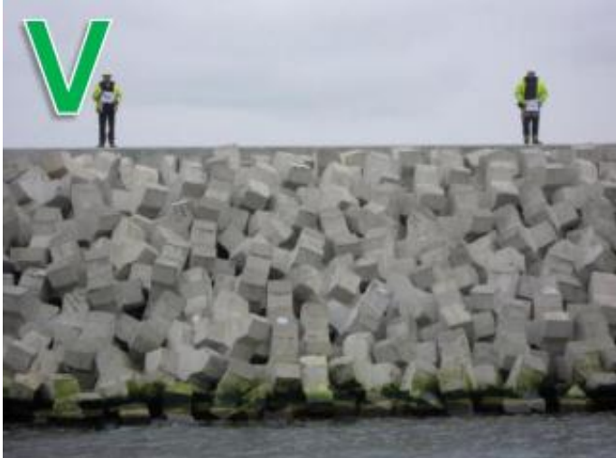
Xbloc random placement: Good packing density
