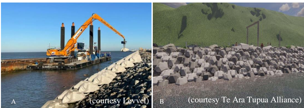
Figure 1 A: normal XblocPlus slope and B) adjusted XblocPlus slope to blend in surroundings
