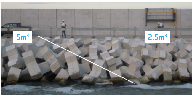
Figure 11-3: Transition between 2 sizes of Xbloc
