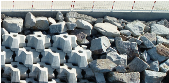
Figure 11-5: Transition between XblocPlus and rock armour
