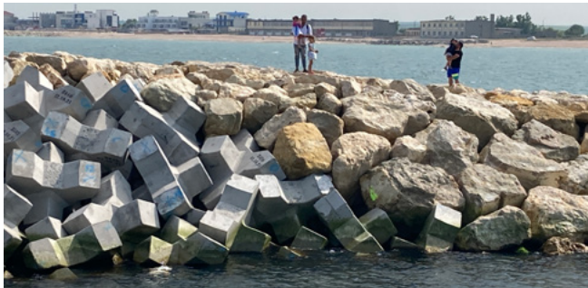
Figure 11-1: Transition between Xbloc and rock armour
