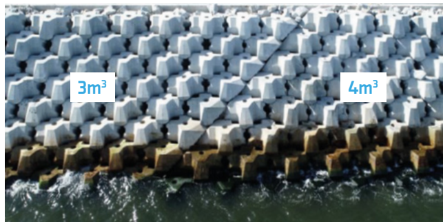
Figure 11-7: Transition with XP-Trans units between different unit sizes of XblocPlus
