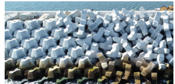
Figure 11-9: Transition between XblocPlus and Xbloc
