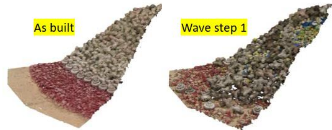
Figure 5: Photo of as-built section of roundhead and damage after test series 1
